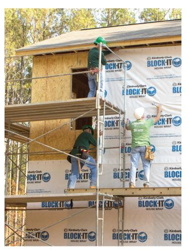
BLOCK-IT\* House Wrap has patented breathable barrier technology engineered to allow water vapor to escape from the wall cavity and to help prevent water damage. It is rated at 15 perms, higher than code requirements.
